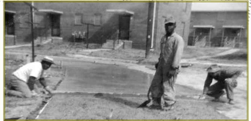
Green Hunter Homes during construction in 1950-51. Photo courtesy of the Black History Society photograph collection. Hall County Library.
